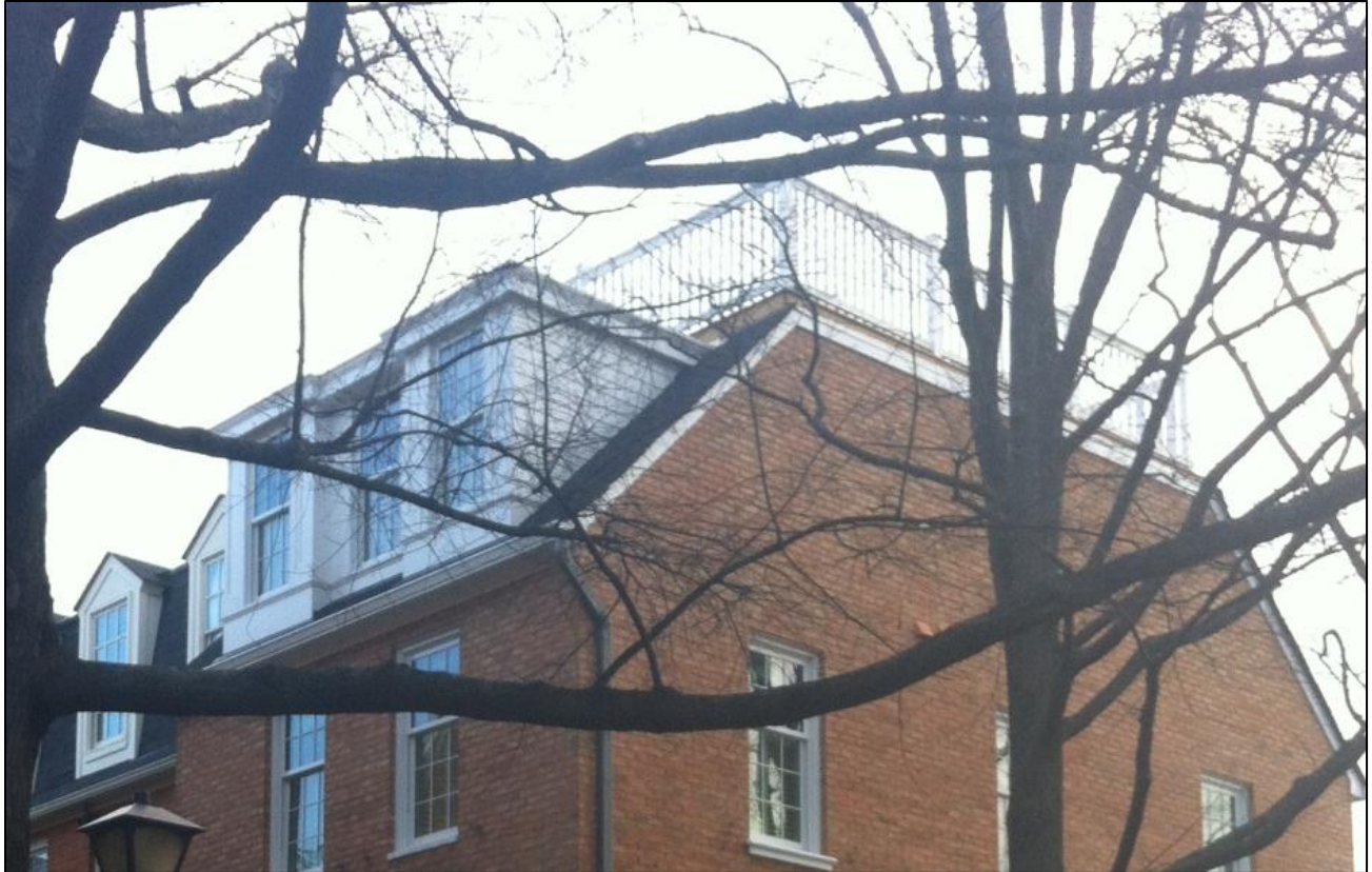
Current Dormer as Constructed
