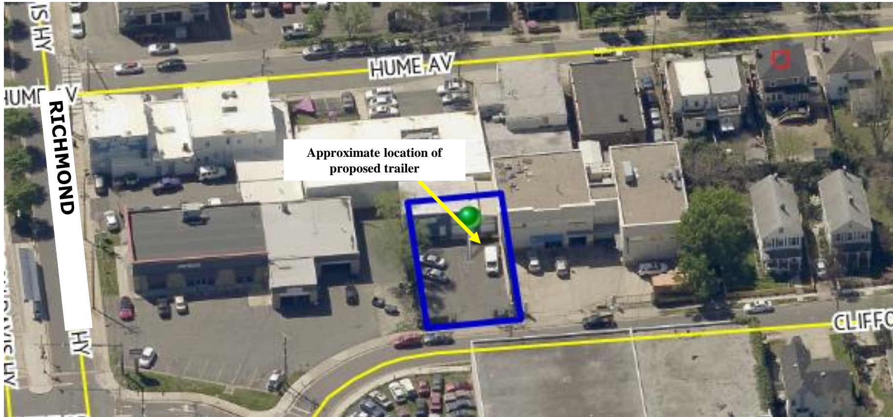
Site Context with Nearby Residential from the north side of Clifford Avenue
