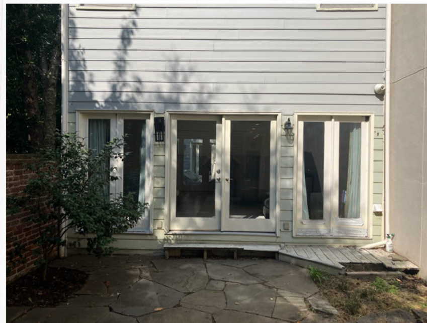
EXISTING PHOTOS - REAR
