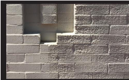
The brick on the right side in the photo has been sandblasted, causing the outer hard fired layer to be removed and making it more susceptible to further damage and destroying its historic architectural character. The Board considers this demolition of the masonry.
