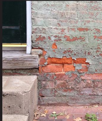
Rising damp (water wicking from below) has caused the face of this early brick to crumble from the freeze-thaw cycle.
