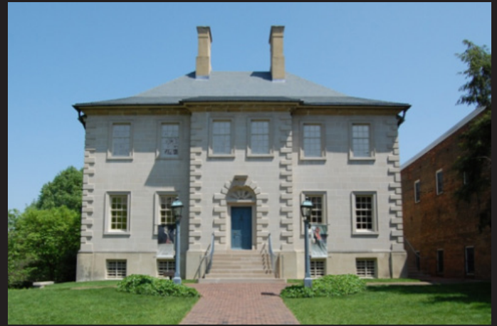
The Carlyle House was originally constructed in the 18th Century with Aquia Creek sandstone.
