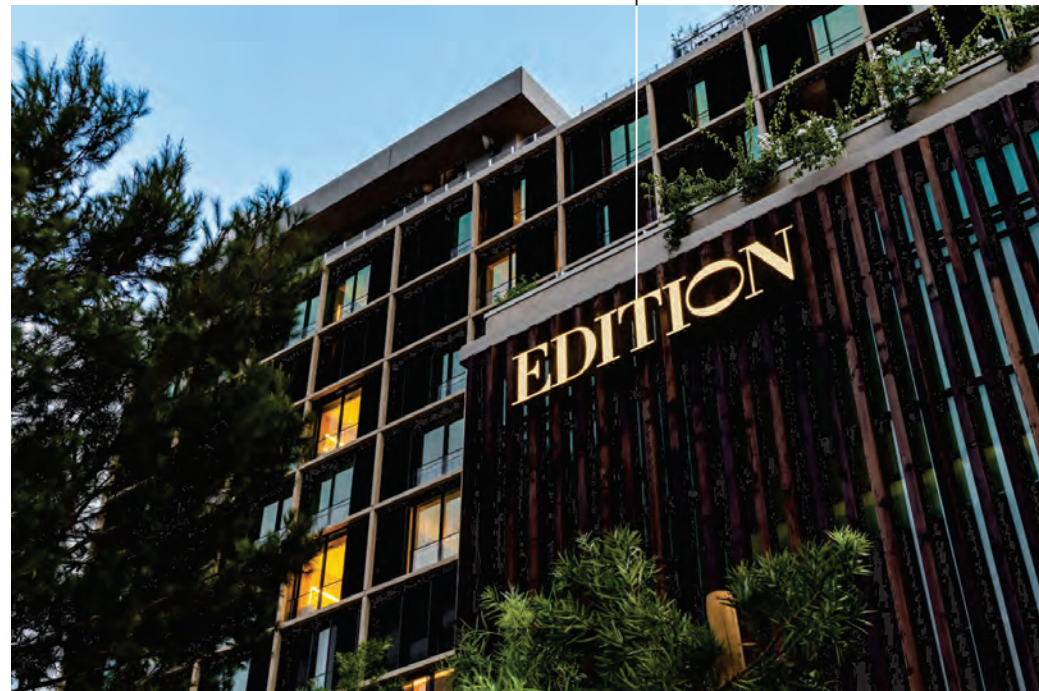
Face Illuminated Channel Letters Mounted to architectural metal rail system
