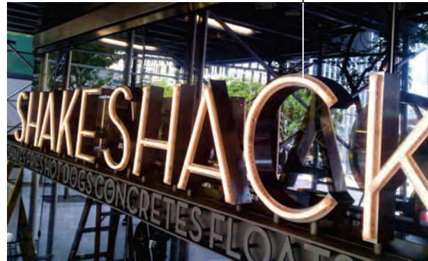
Push-thru acrylic face Illuminated Channel Letters Mounted on structural architectural rail
