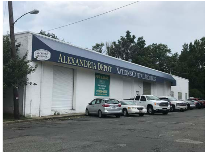
Figure 2: Existing building - Fannon Street facade.
