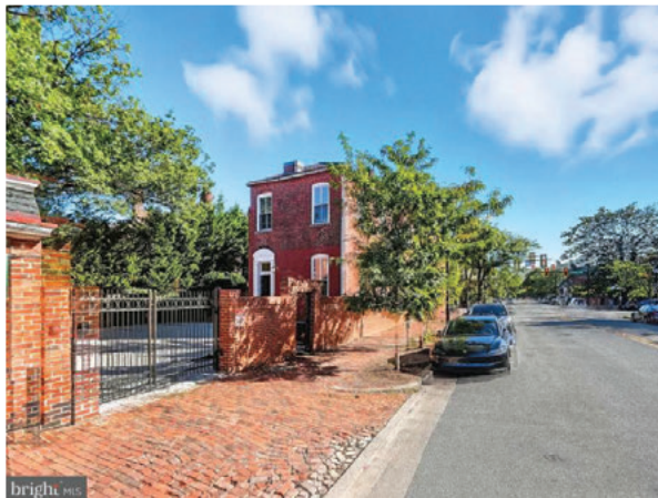
Existing Frontage Wall and entrances from Columbus: 6' brick wall with gated driveway and 3' 6" walking gate, including archway
