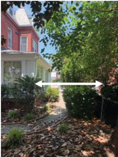
View from Prince St along the East side of the house into back yard, 11' opening per the Plat
