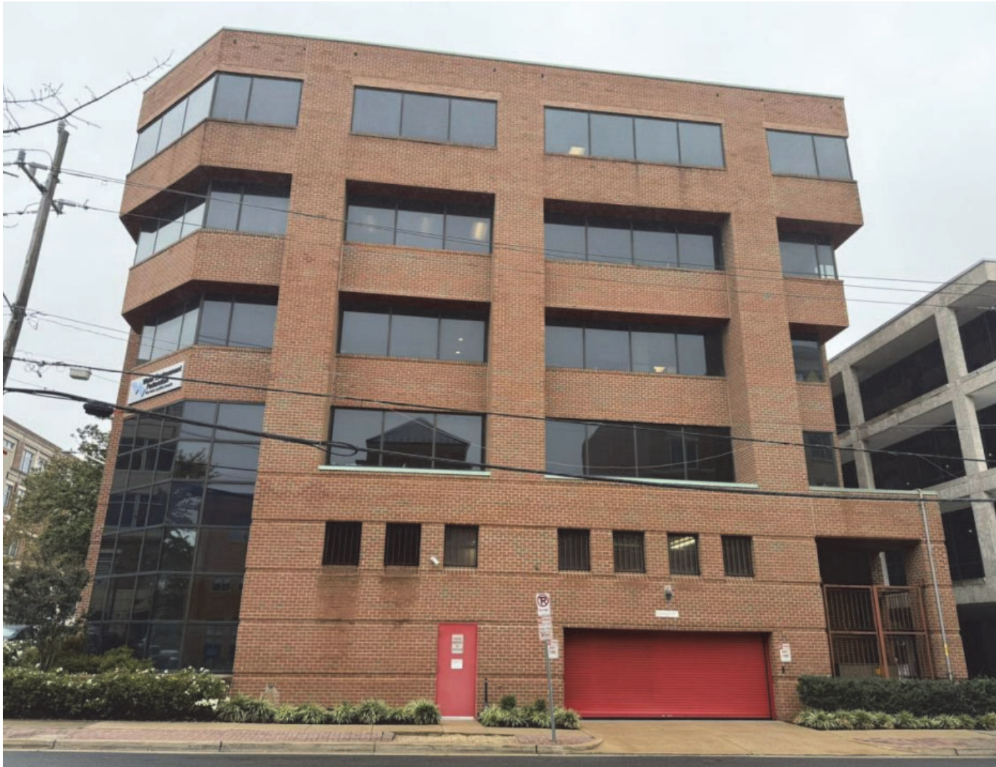
N. ST ASAPH STREET (EAST FACADE)
