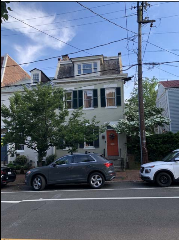
514 PRINCE STREET - OLD & HISTORIC ALEXANDRIA
