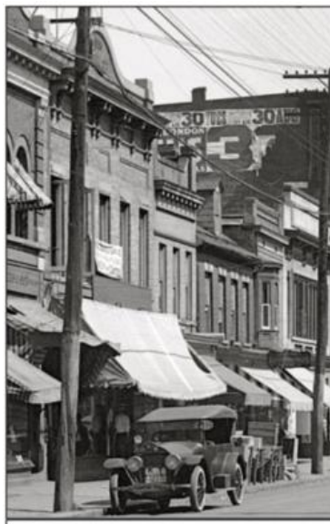
Photo 1: The original two buildings located at 615 King Street site (c.1921)
