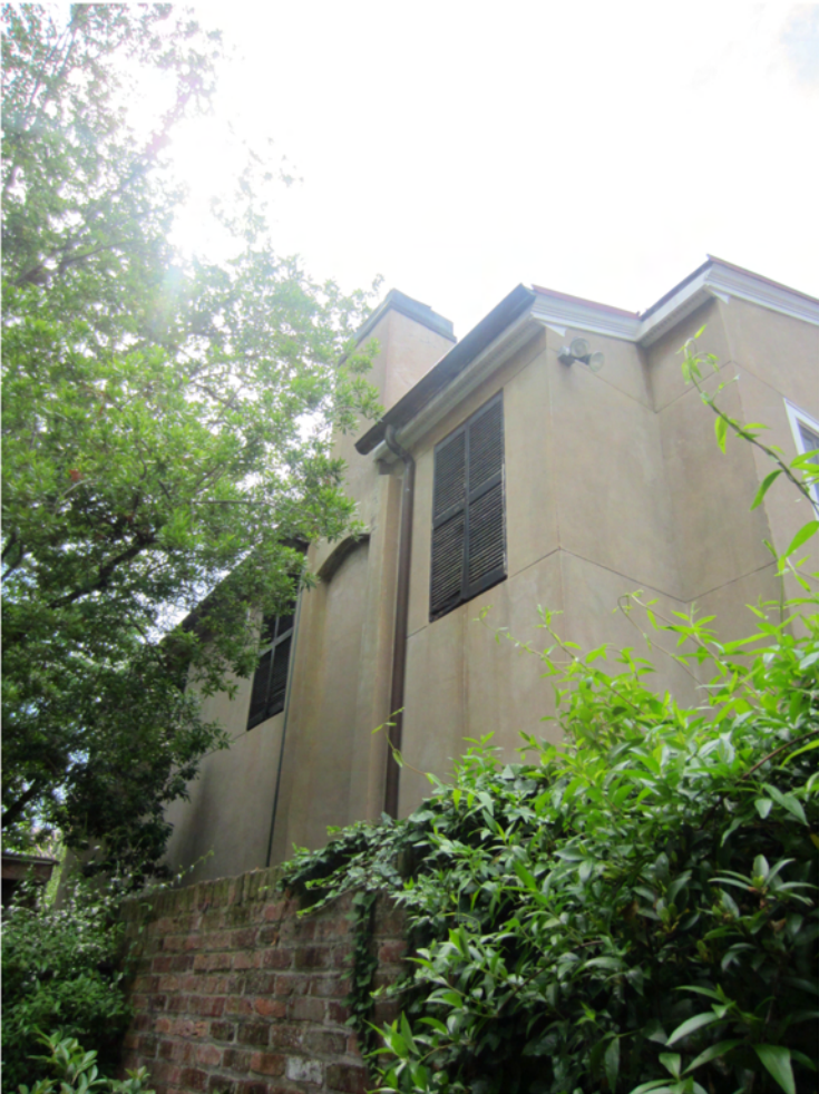
3. Blind wall of 207 S. Fairfax to South.
