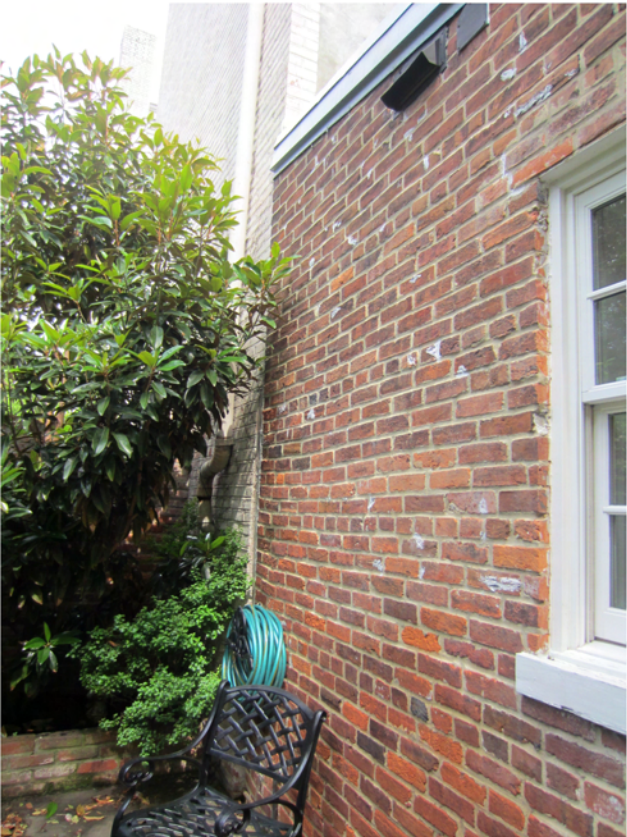
2. South wall of 1-story Ell- looking South
