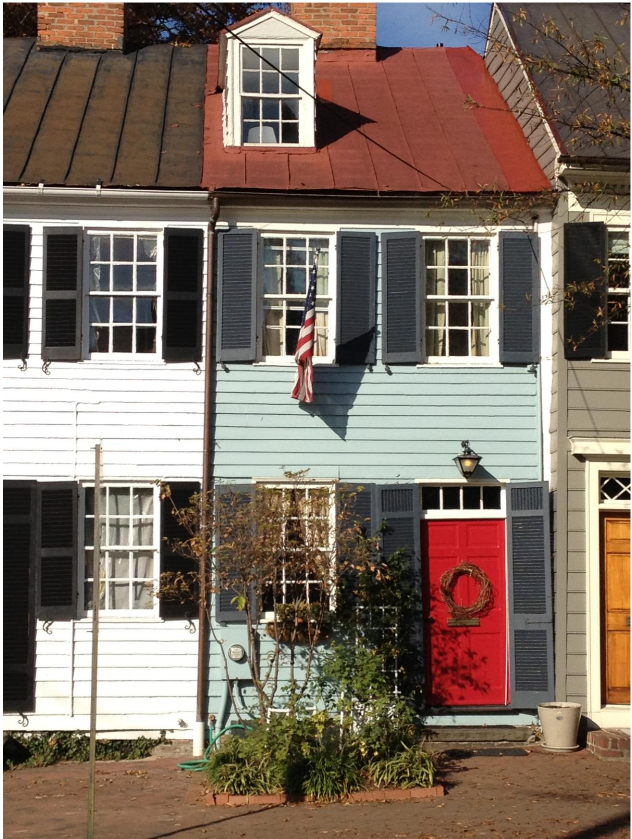
Front Façade – 323 Duke St.
