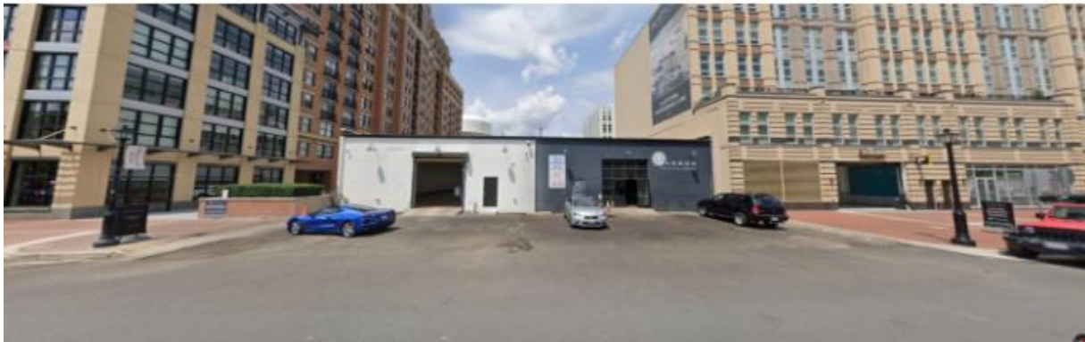
Figure 4: As part of a separate City Council lease agreement review, a new sidewalk section in front of Yates Auto Care will provide continuous and safe pedestrian passage along the 1000 block of North Fayette Street.
