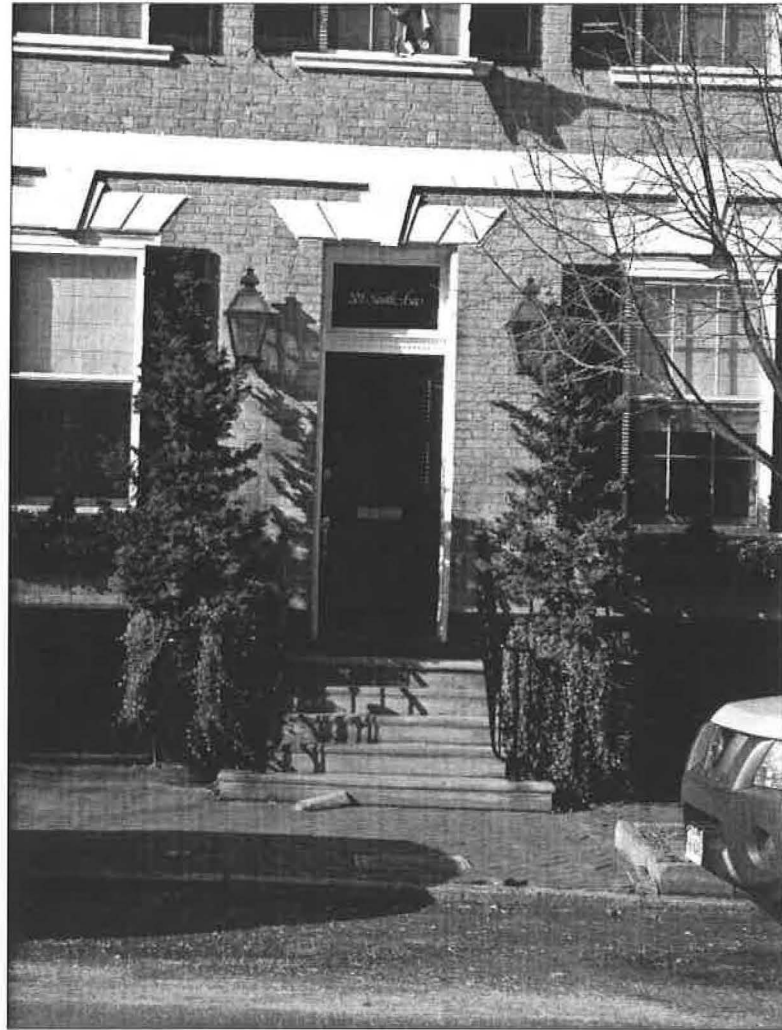
Front door facing S. Lee Street. Note brick jambs altered for a lessened-width opening.
