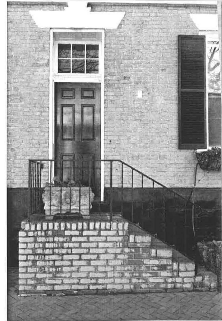
Abandoned door and stoop on Prince Street. Note brick jambs altered for a lessened-width opening.
