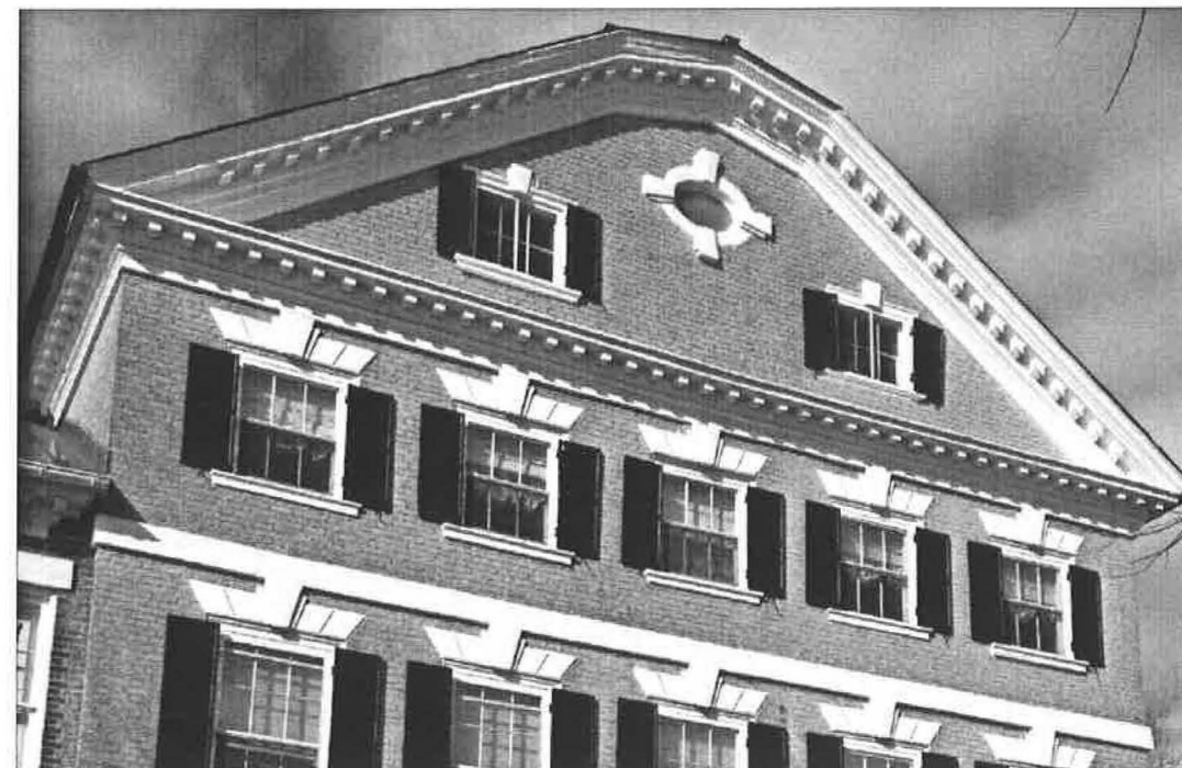
Detail of east gable
