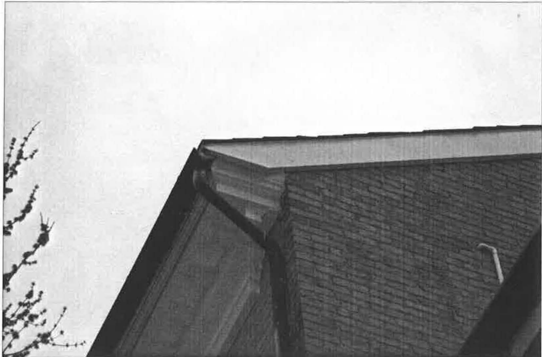
Cornice Detail @ northwest corner
