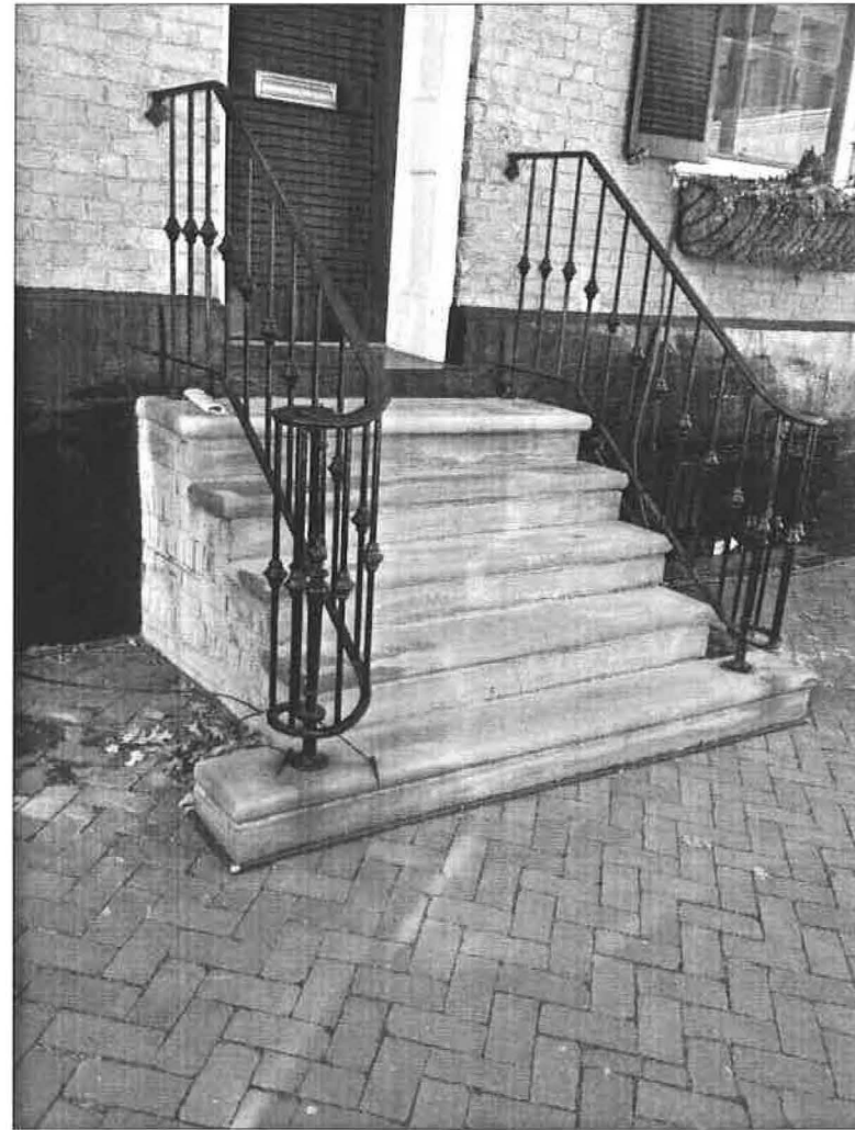
Modern steps and rail at front door.
