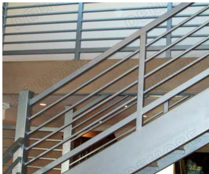
Example of a square aluminum balustrade.
