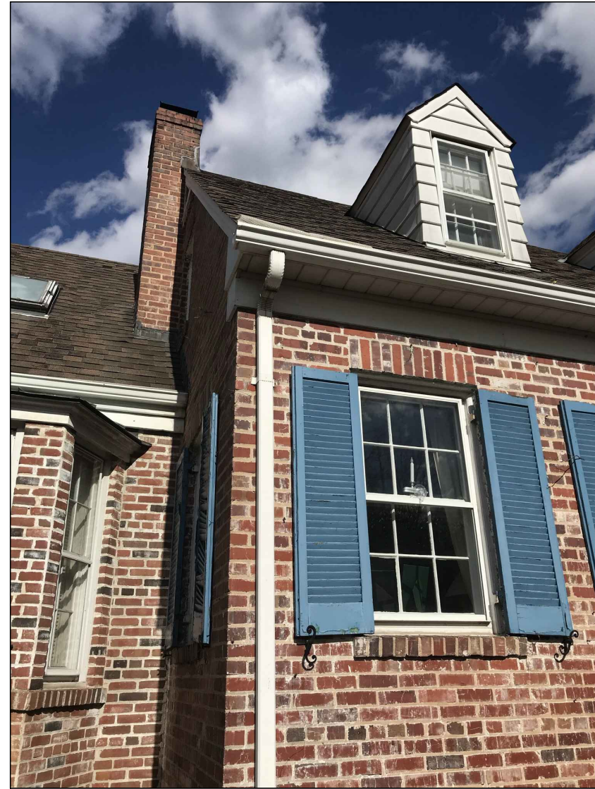
1940 original gable dormer
