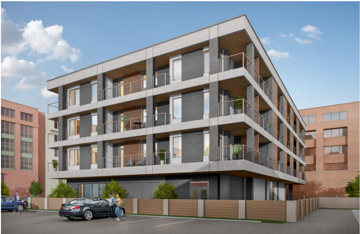
Figure 5: View of northwest corner of building
