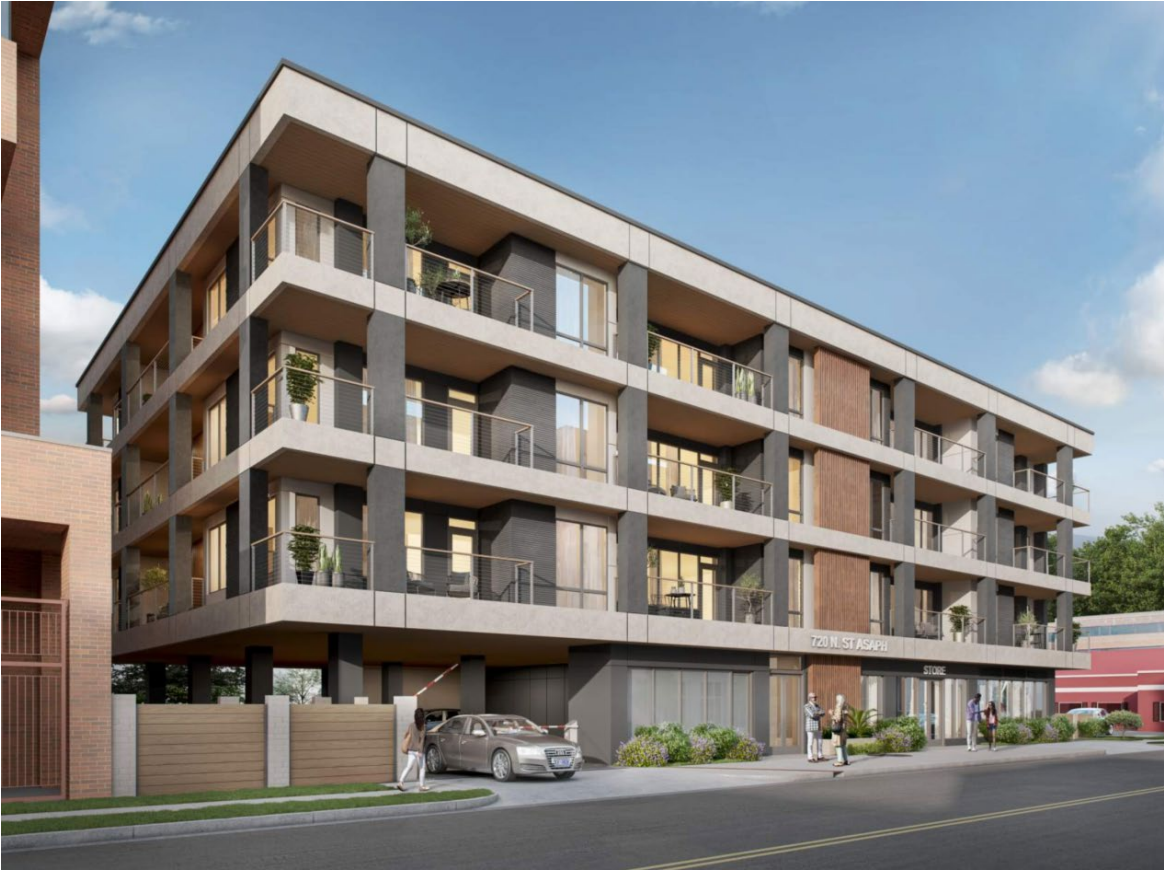
Figure 4: View of southeast corner of building
