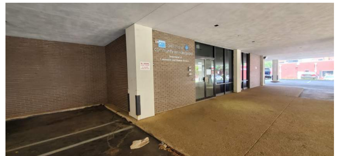
EXISTING BRICK FINISH
