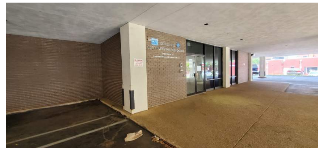
EXISTING BRICK FINISH
