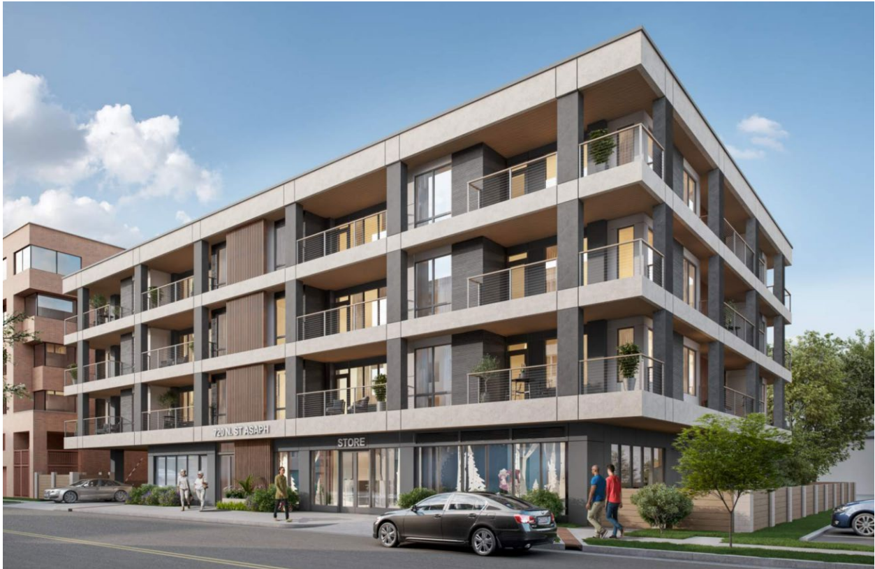
Figure 3: View of northeast corner of building
