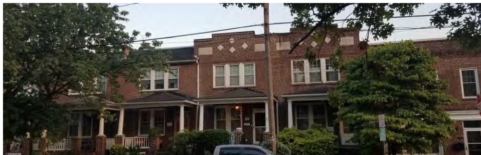
1400 block of Cameron Street (south side) directly across from Jefferson
