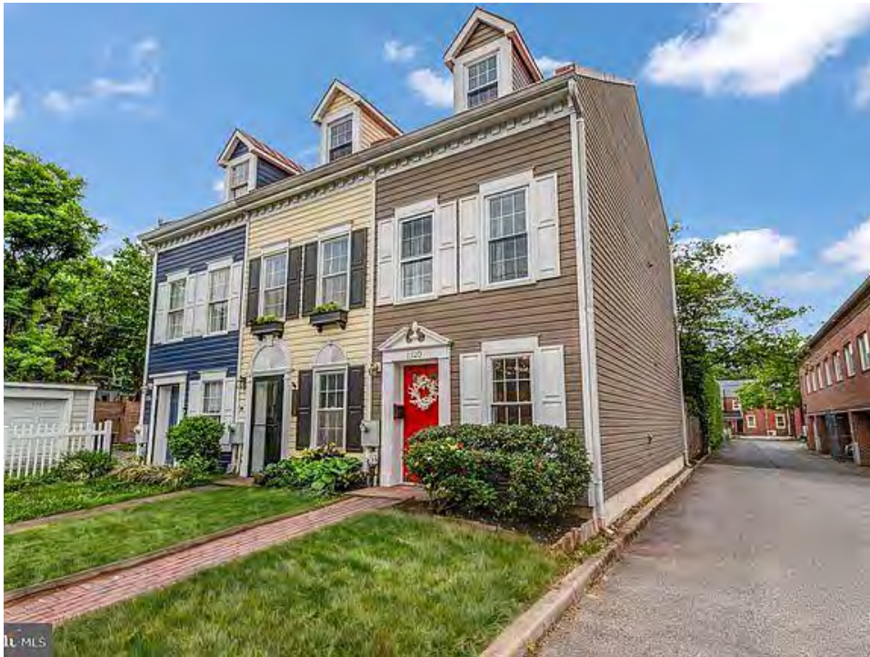
1300 block of Cameron Street (south side) directly adjacent to the site
