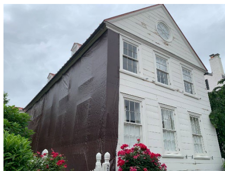
Figure 1. The siding on the south elevation has been removed.
