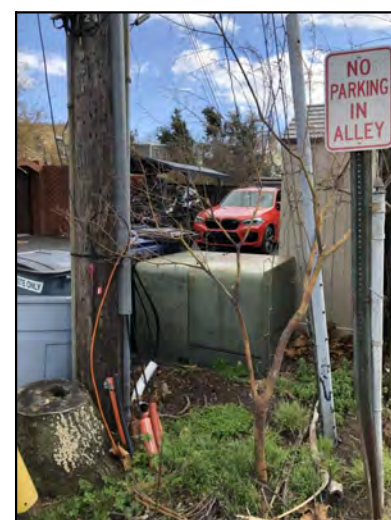
2D - VIEW OF NORTHWEST CORNER LOOKING NORTH
