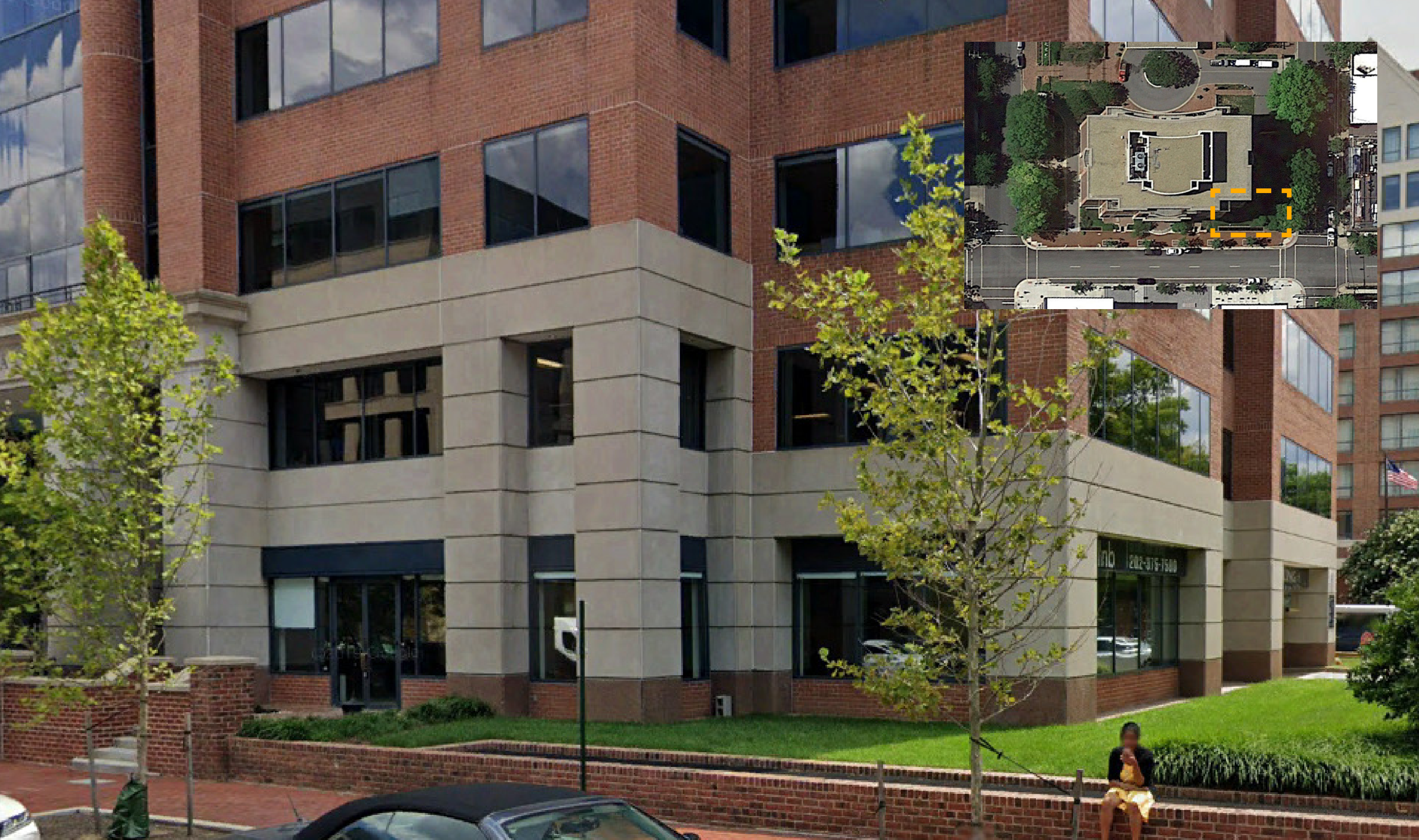
EXISTING NW CORNER
