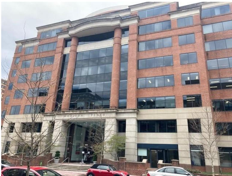
Figure 1- Existing Office Building from Montgomery Street
