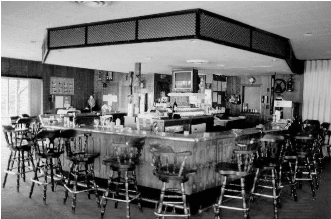
Figure 29: 1995 View of the Second-floor Bar Before Renovation
