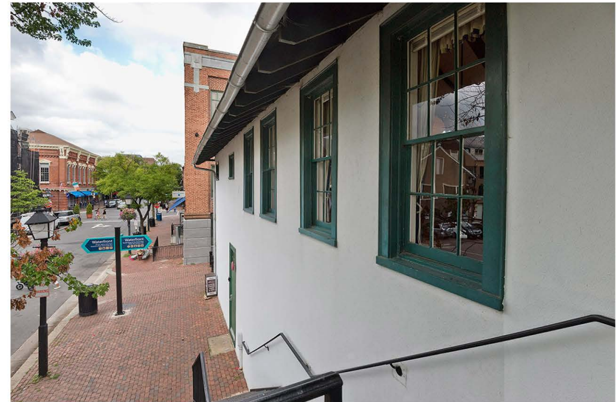
SOUTH ELEVATION FROM UPPER FLOOR PORCH @ KING STREET
