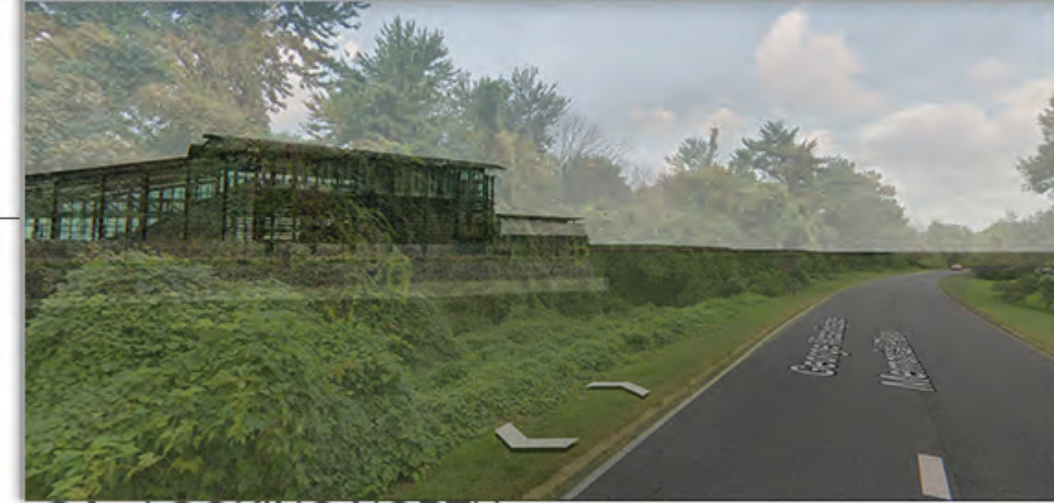
C1 - LOOKING NORTH
