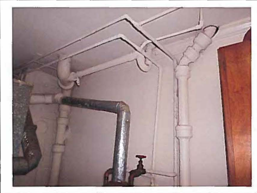
7 View of piping and exposed ductwork at interior.
