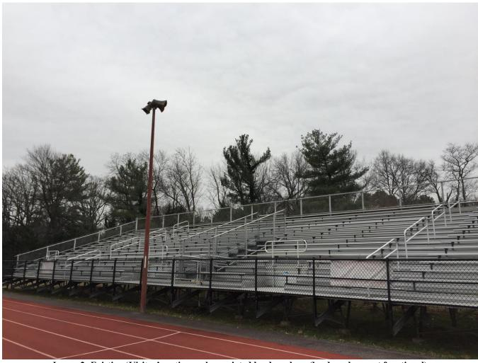
Image 2: Existing 'Visitor' seating and associated loudspeakers (loudspeakers not functional)
