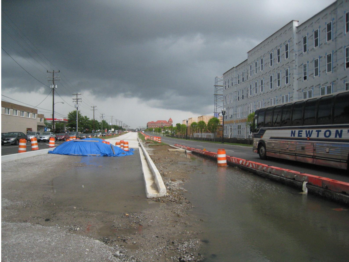
Figure 2 – Ongoing Construction of the Transitway
