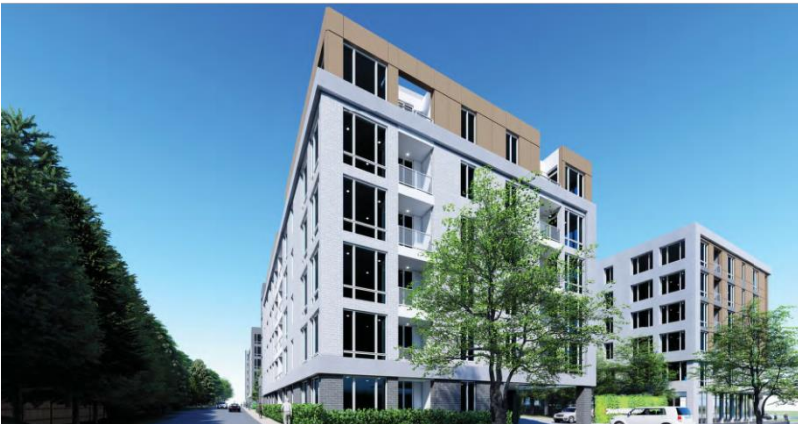
Rear of west wing, from Mark Center Drive.
